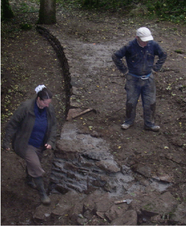
The permanent dam - September 2013.
