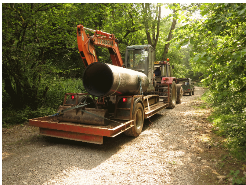
Digger and piping being transported to site - July 2013.
