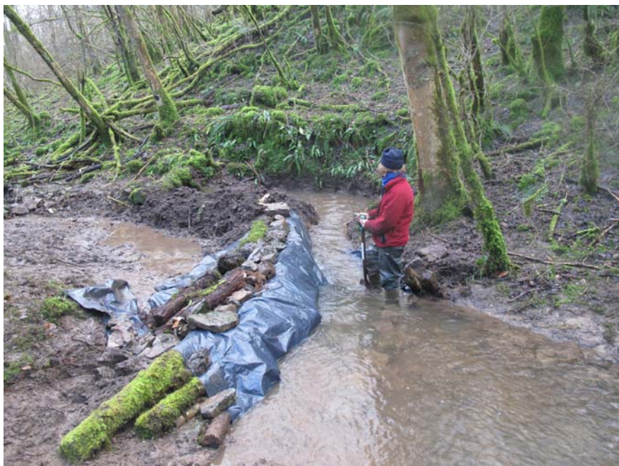
The first temporary dam at Longwood Valley Sink.
